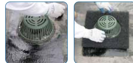
Apply adhesive to secure Filter to roof. Use Roofing Cement on asphalt membrane. Use water-based adhesive to secure to synthetic roof membrane.
