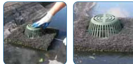
Insert a 1/8" metal rod horizontally through Roof Drain Filter and strainer.
