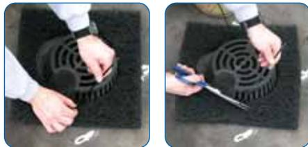
Push a cable tie down through Filter Media an inch from center cut out. Bend tip of cable tie back on itself firmly and insert into strainer, loop around strainer fin and pull back out to attach. Needle nose pliers may be helpful to grab cable tie end to pull back through strainer. Pull zip ties snug to secure Filter to drain.
