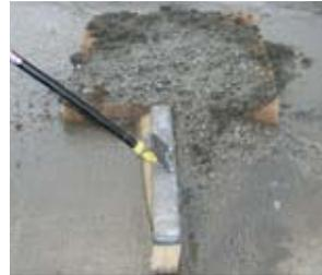
**1. Remove sediment** from the sides of the filter by sweeping away from Inlet Filter.
