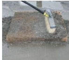
**2. Remove sediment** from the top of the filter by sweeping off of Inlet Filter.
